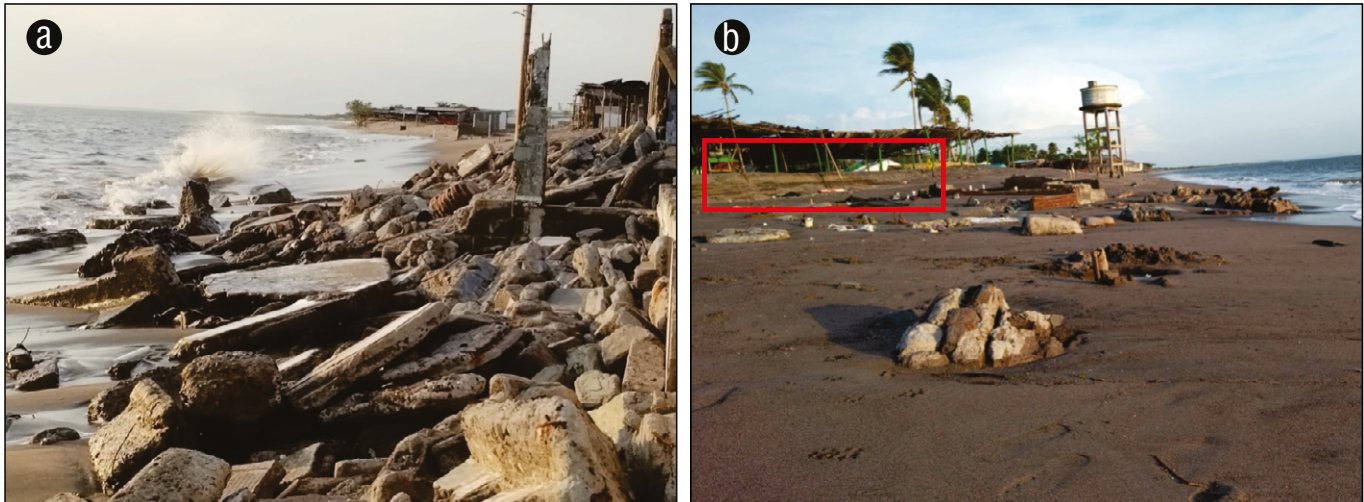
Figure 8. Impact of sea level rise on the coastal infrastructure of Cedeño, Pacific coast of Honduras (PCH). Submerged infrastructure due to sea level rise (a) and coastal erosion labeled in red and local businesses destroyed by sea level rise (b).
